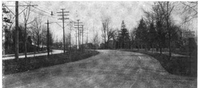
SECTION OF NEWTON BOULEVARD TREATED WITH TARVIA.
